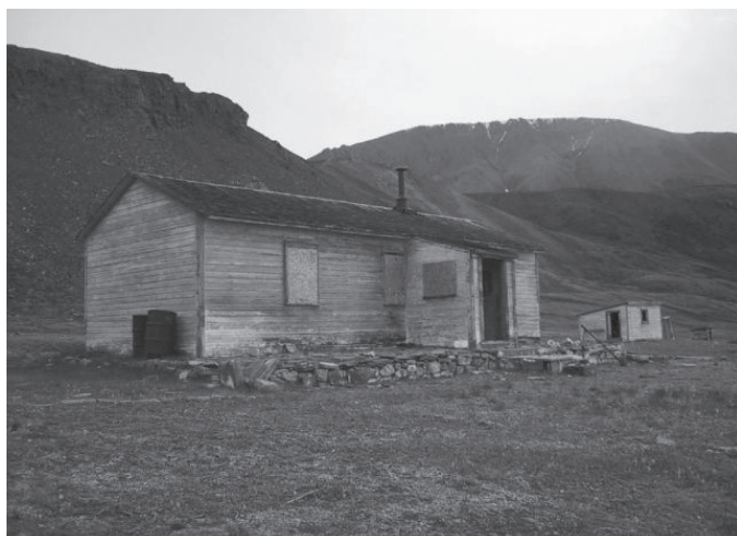
Deserted RCMP building, Dundas Harbour (D.Riedel, 2007) 12
